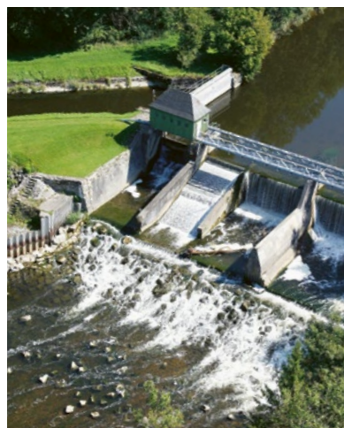
Our water power plant.
